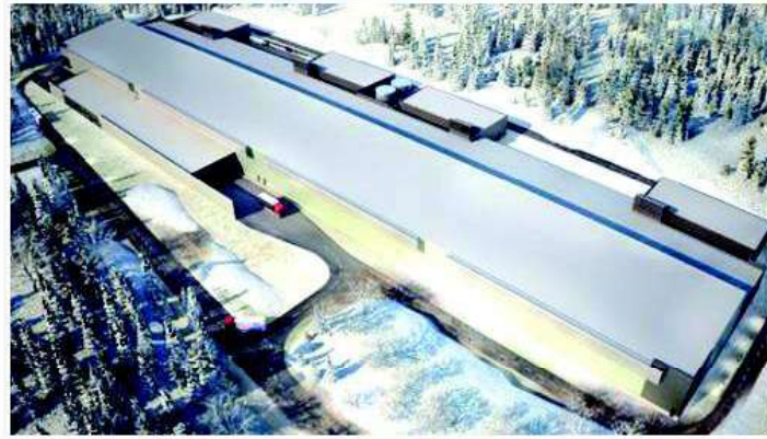
Fig. 2: Data Center near Arctic Circle
